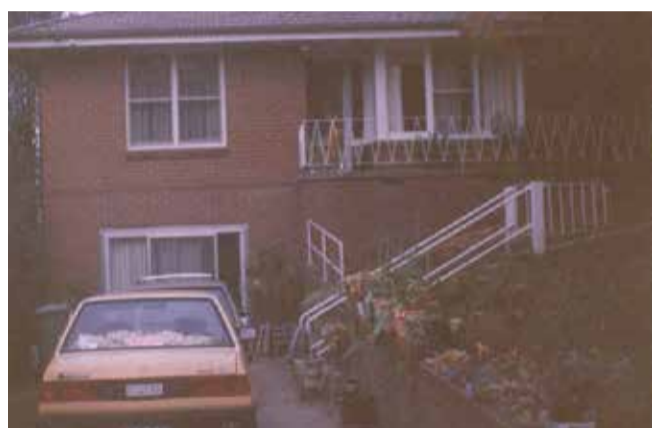
Southern Vale Homes first office
